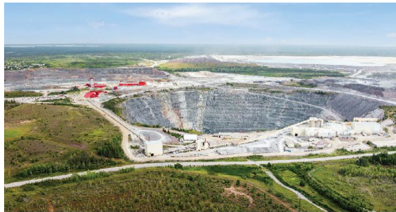
Discovery's existing 15,000 tpd Dome Milling Complex
