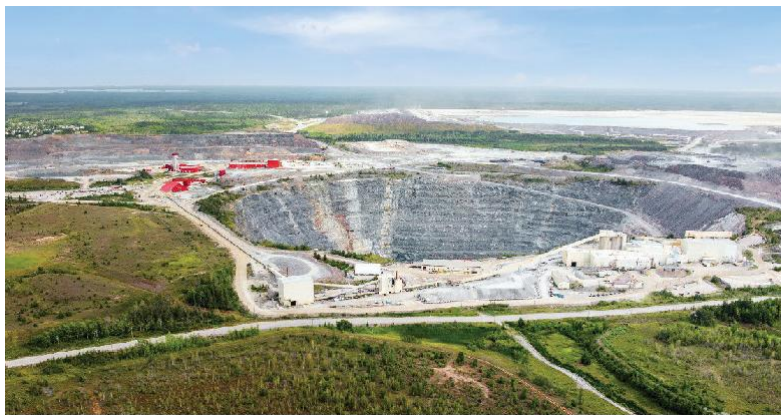
Discovery's existing 15,000 tpd Dome Milling Complex
