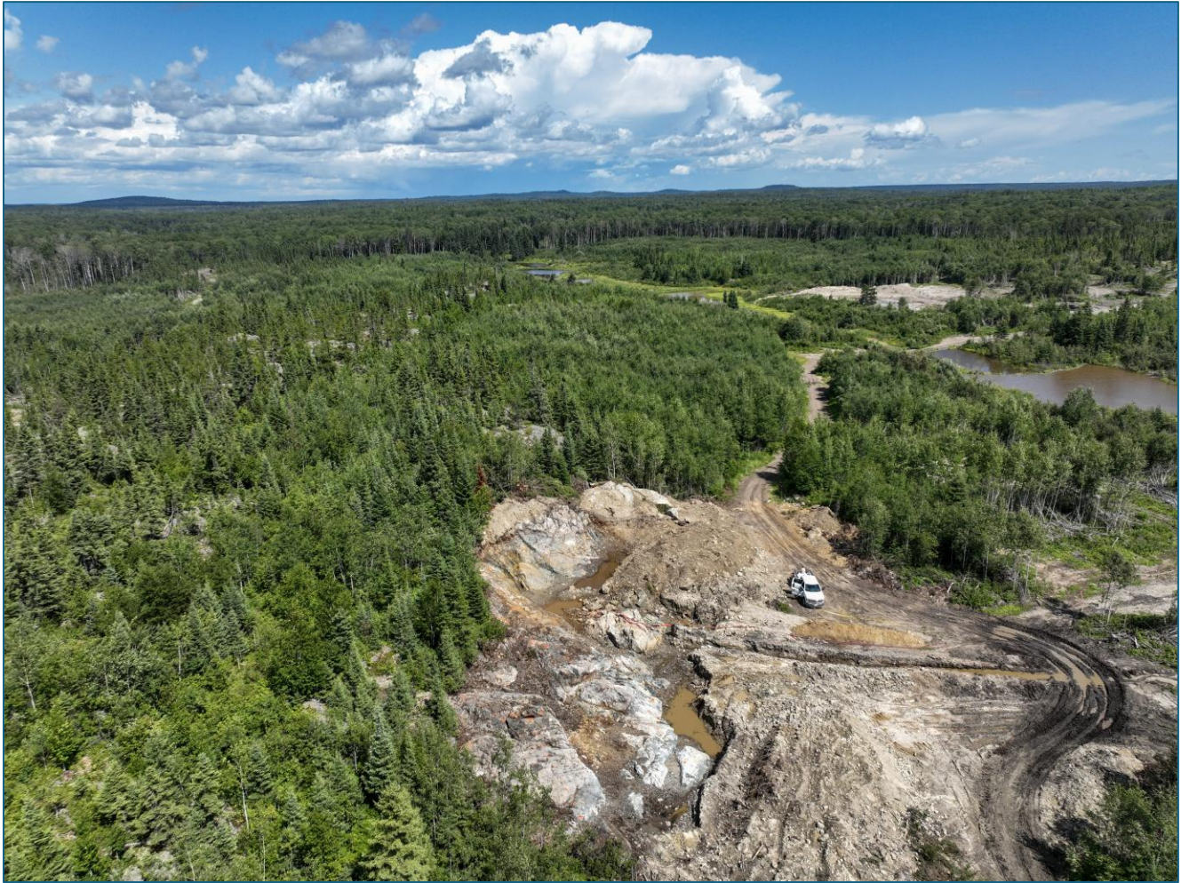
Figure 3 – Recently Completed Trench at Argus West – Looking East Towards Argus North and Argus Main
